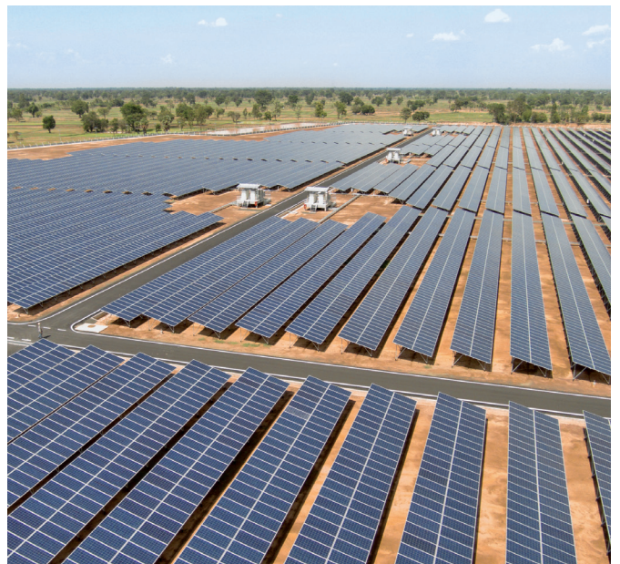
Power conversion skids installed at the solar farms
