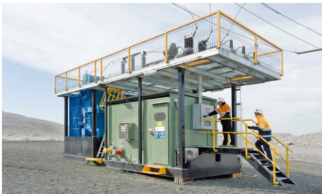
A typical relocatable substation used in above ground mining applications
