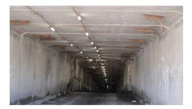
The LED AlphaLite Max is available in 18W and 36W versions, producing equivalent light to a single 36W and 2x36W fluorescent lamps respectively.
